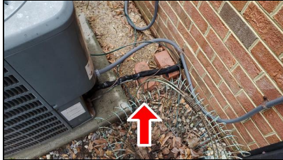
8.5 Item 3(Picture) Example/ Sample- exterior at or near the condenser unit
