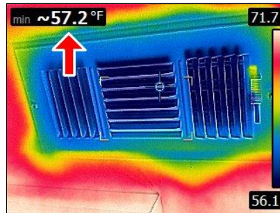
8.0 Item 2(Picture) Example/ Sample- second level air conditioning supply at time of inspection
