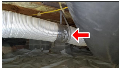
9.4 Item 2(Picture) Appears functional at time of inspection
