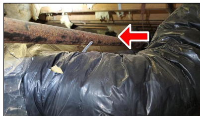
6.7 Item 2(Picture) Example/ Sample- crawlspace
