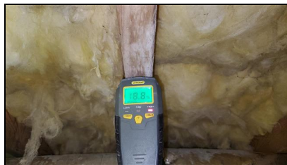
5.0 Item 4(Picture) Example/ Sample- primarily the addition area elevated wood moisture content(WMC) 18% +/- , and fungi
