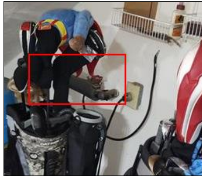
6.2 Item 2(Picture) additional water cutoffs located in garage
