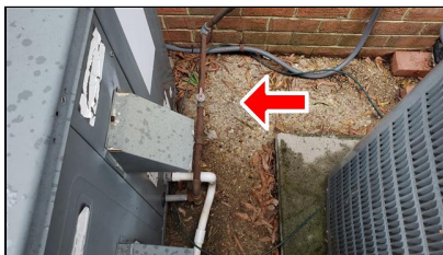
6.7 Item 1(Picture) Example/ Sample- rear of home
