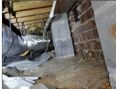
5.0 Item 10(Picture) Example/ Sample- rear of the home
