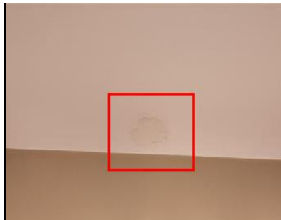
3.0 Item 1(Picture) Example/ Sample- Second level Hall Bathroom
