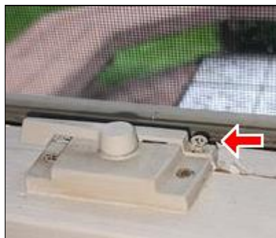
3.5 Item 3(Picture) Example/ Sample- Sunroom- Loose hardware
