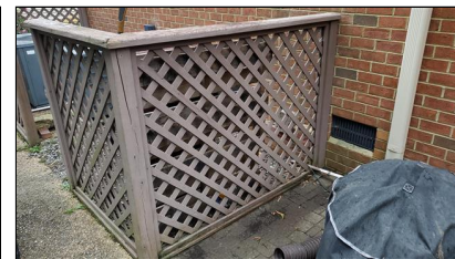
2.2 Item 2(Picture) Example/ Sample- rear of home
