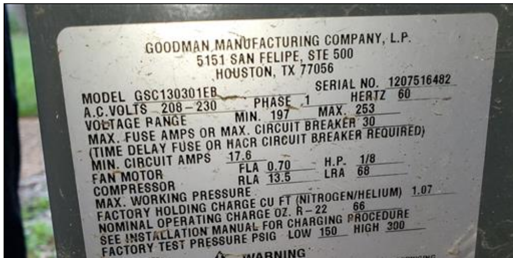
HVAC condenser label – located at the rear of the home – GOODMAN MANUFACTURING – manufacturer year 2012
